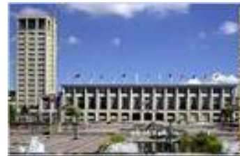
City of Havre (France)
